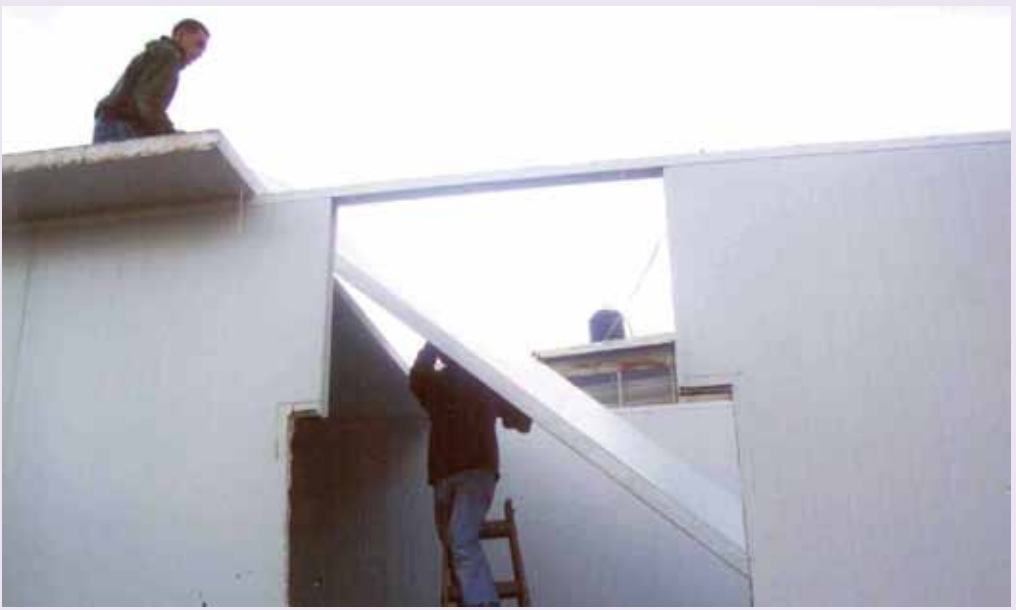
Figure 10: The self demolition of the house of UA / Source: Al-Maqdese Archive.
