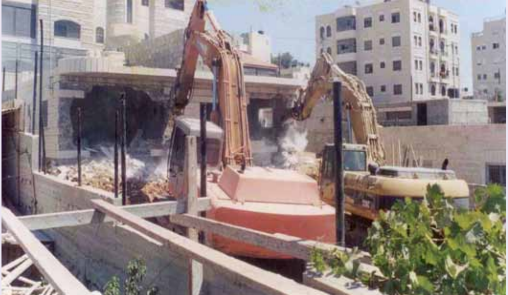
Figure 7: The destruction of the home of Rehab Moustafa Al-Jabri./ Source: Al-Maqdese Archive.
