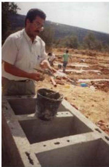
Installing a Grey Water Garden in Brouquin
