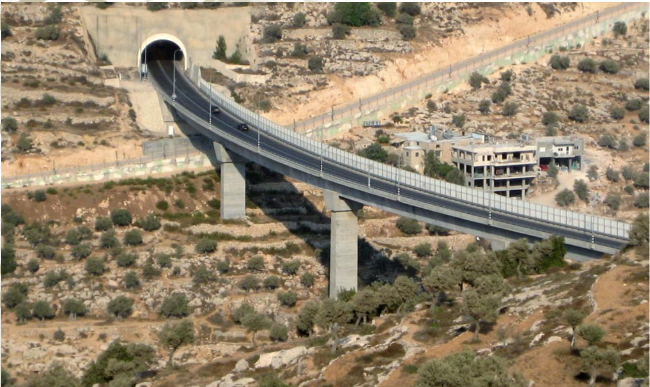
Bypass road 60 (Tunnel)
