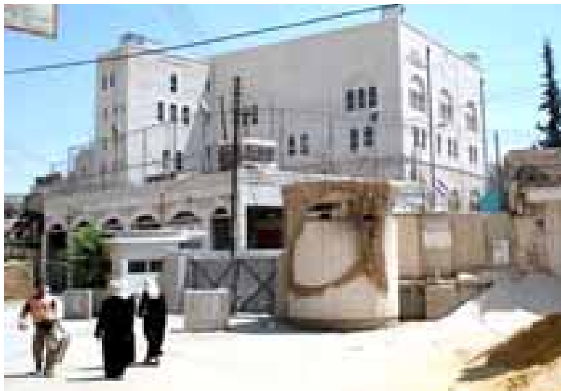
Palestinians passing in front of Israeli settlement [originally Palestinian building] in H2
