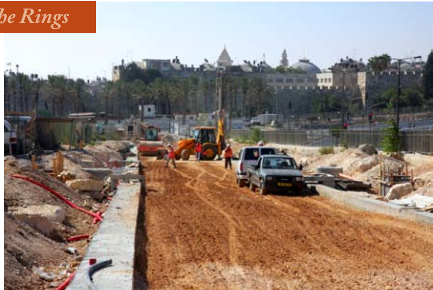
Construction of the Jerusalem Light Rail Project
