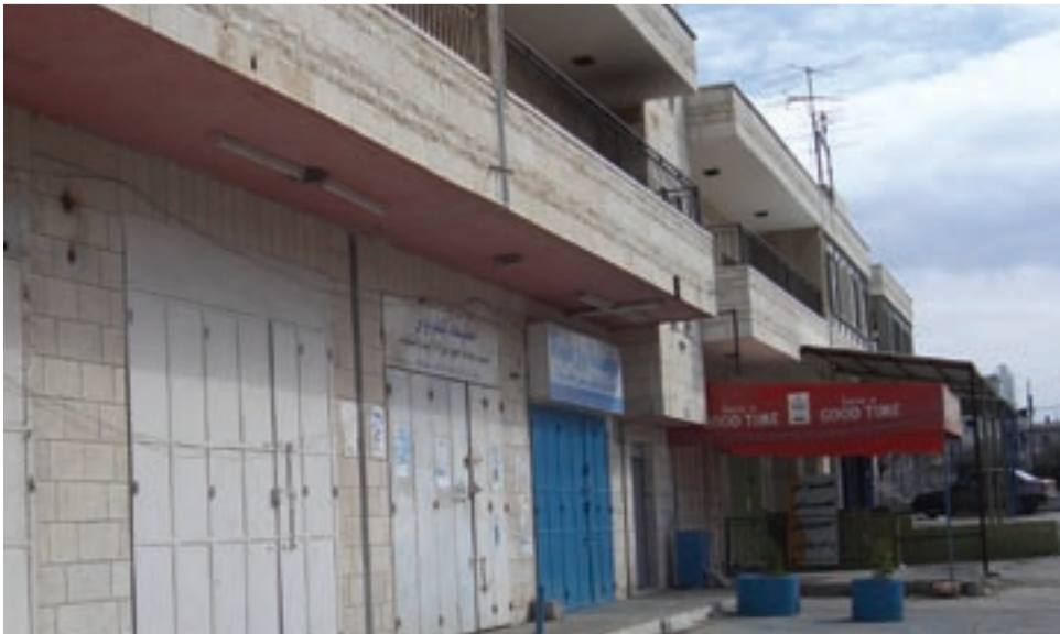
Shops have been boarded up as businesses desert the area.
