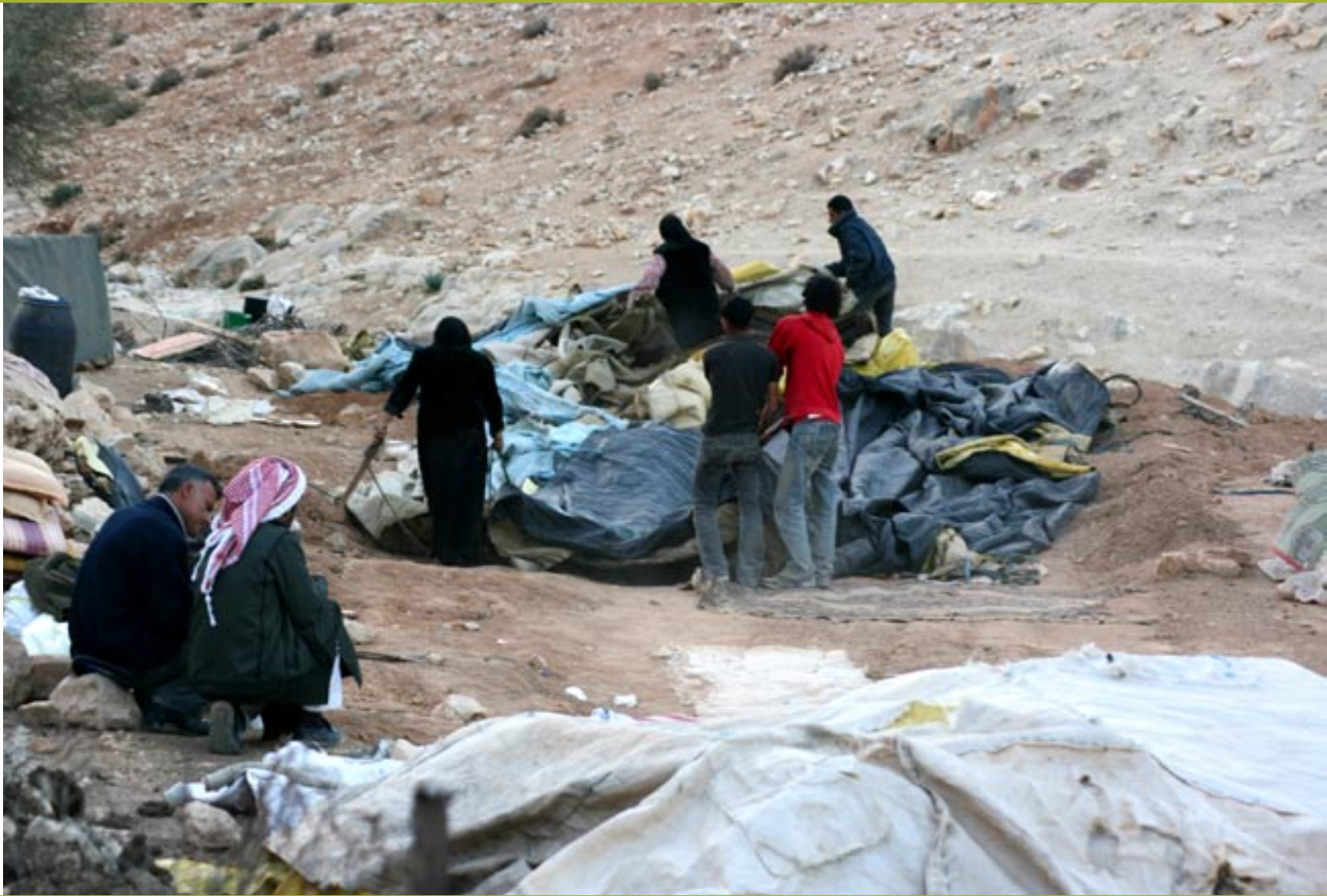
Destruction of Palestinian homes near Abu George Junction.
