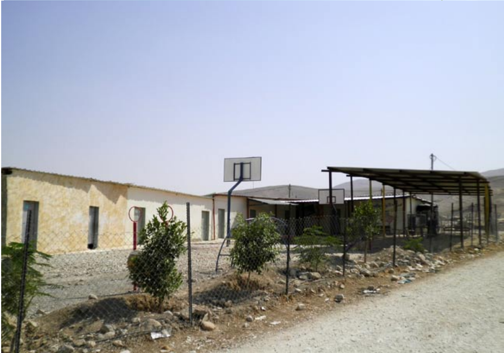
Fayasel al Fuqa school built by MA'AN and funded by the Norwegian Representative Office and Pal Tel.
