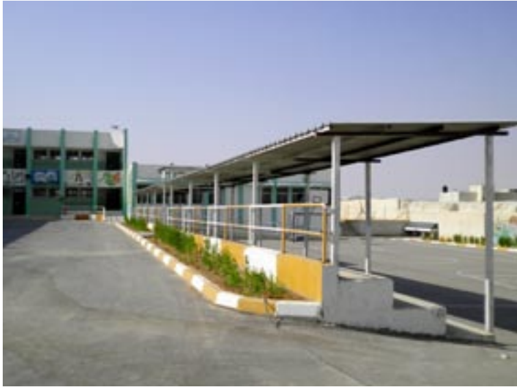
Sunshield installed by MA'AN in a Jordan Valley school
