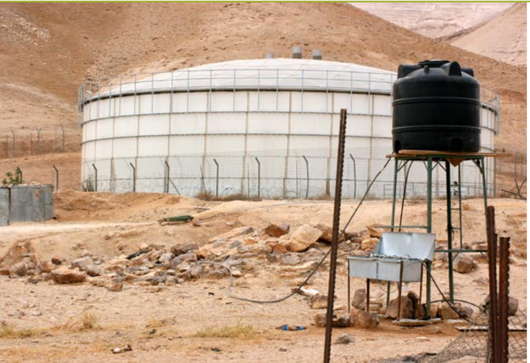
A 2000 m 3 water reservoir for the Israeli Settlement of Araya
